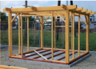
Timber frame construction
