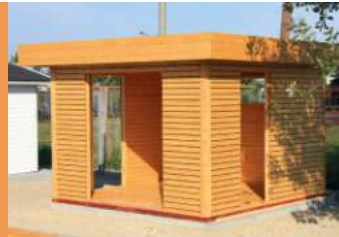
Roof boarding and wall cladding
