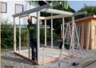
Assembling the skeletal structure
