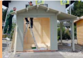
Constructing the roof boarding
