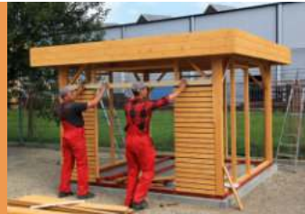
Mounting the rhombus cladding
